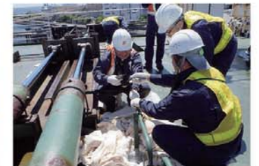
Parts replacement for prevention of oil spill
